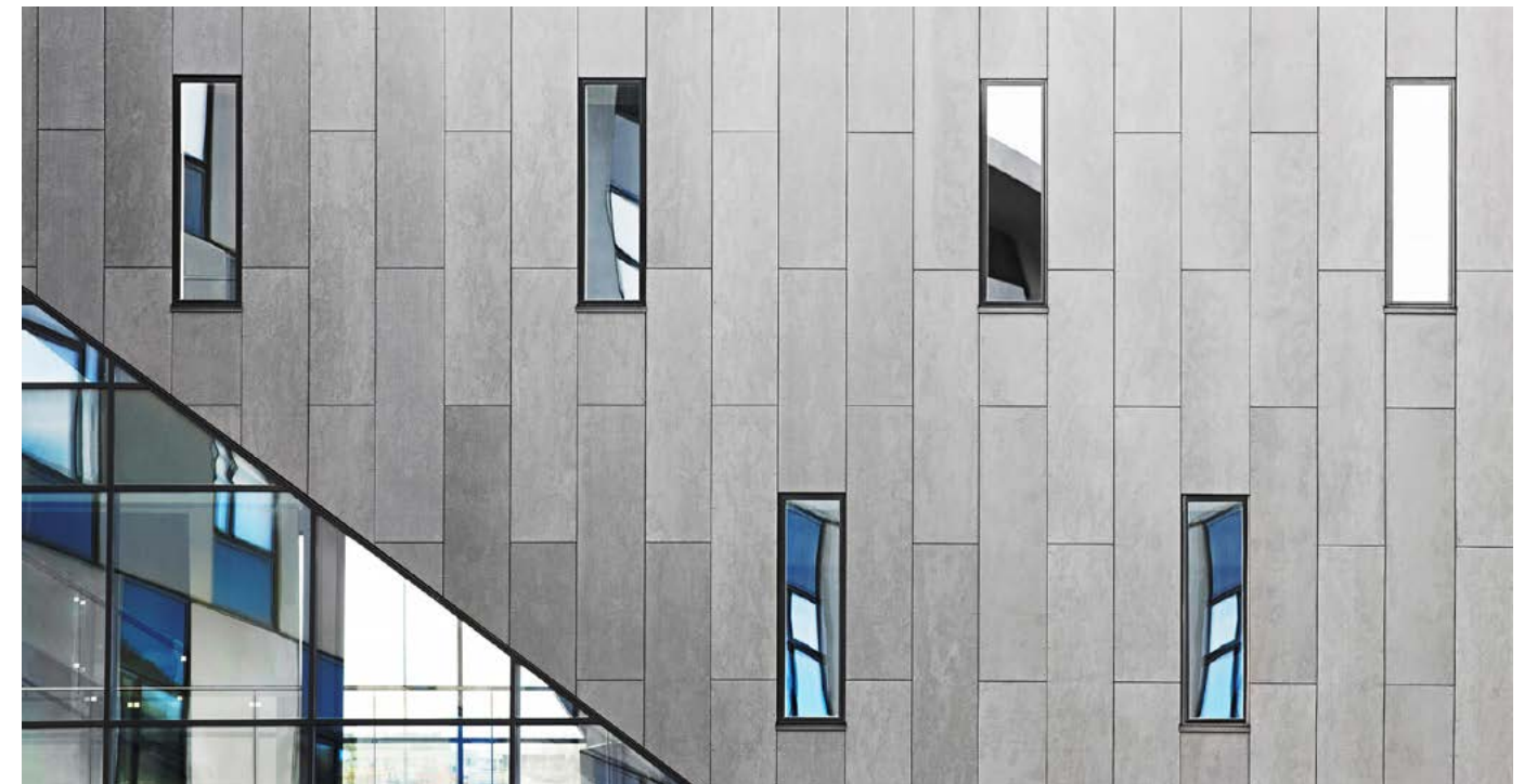
The Vision house, Ålborg, Denmark. Architect: KPF arkitekter, Ålborg, Denmark. Builder: C.W. Obel Ejendomme A/S, Ålborg, Denmark.
